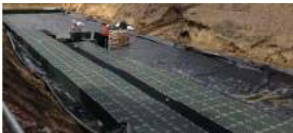
A storm water tank has been installed and we are progressing with the installation of the site haul road.
